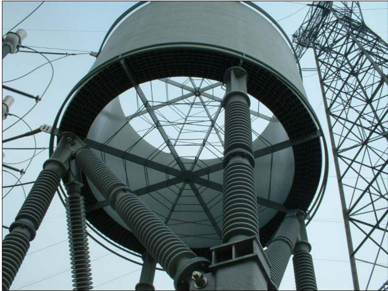
Typical Air-Cooled Reactor
