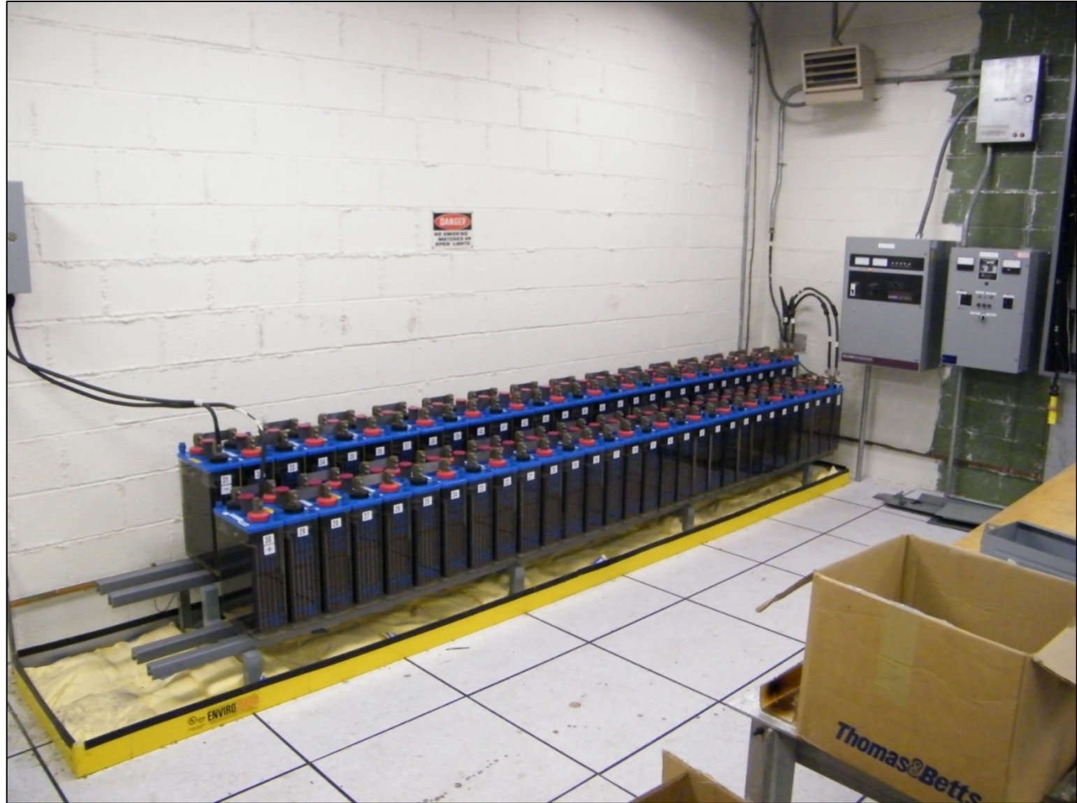
Battery Bank in a 500 kV Substation
