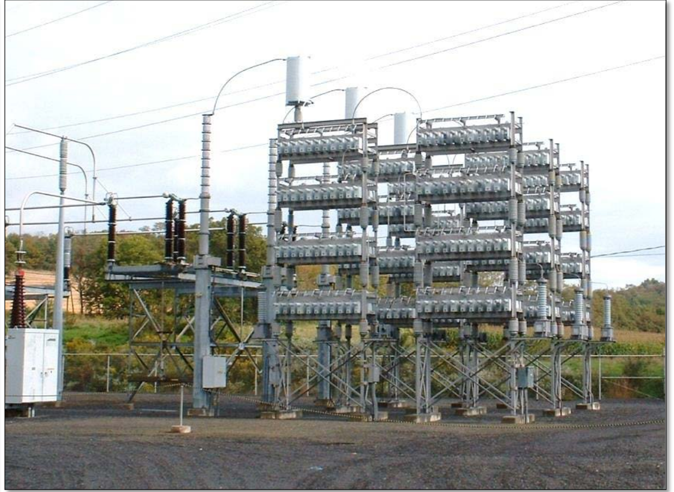
230 kV Capacitor Bank
