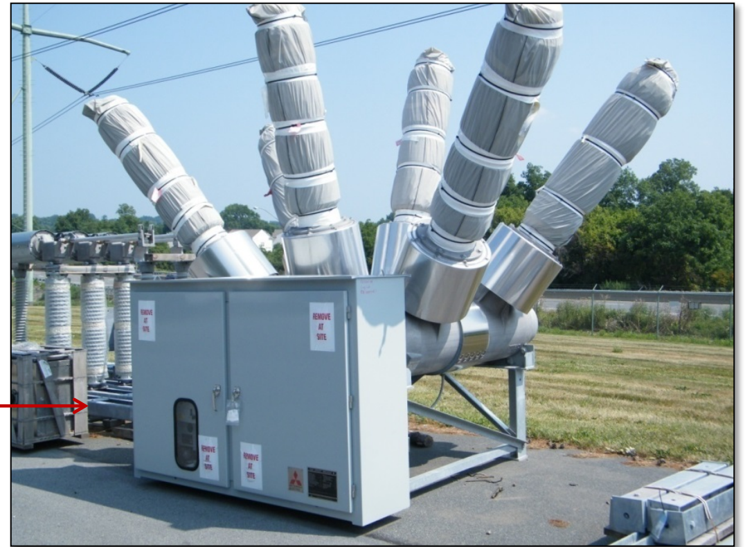
230 kV SF-6 Circuit Breaker
