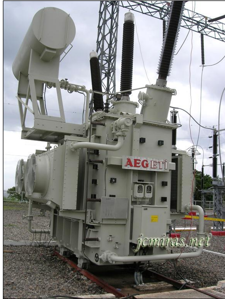
Oil-Cooled Shunt Reactor
