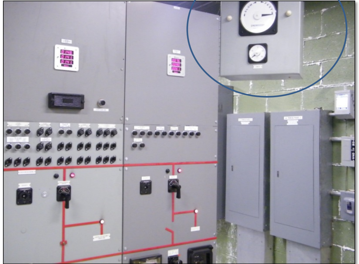
Control Panel with Synchroscope
