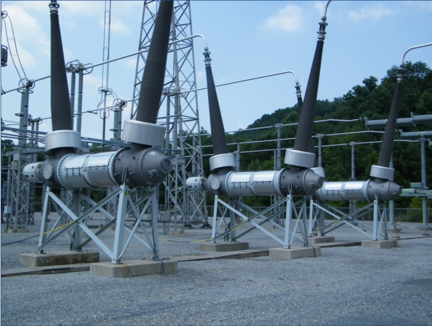
500 kV SF-6 Circuit Breakers
