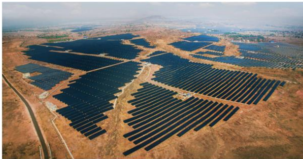
Topaz Solar Farm, San Luis Obispo County, California
