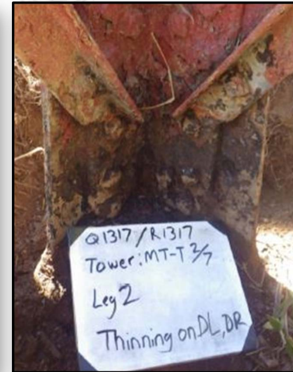
Figure 1: Examples of 25-30% foundation structure loss
