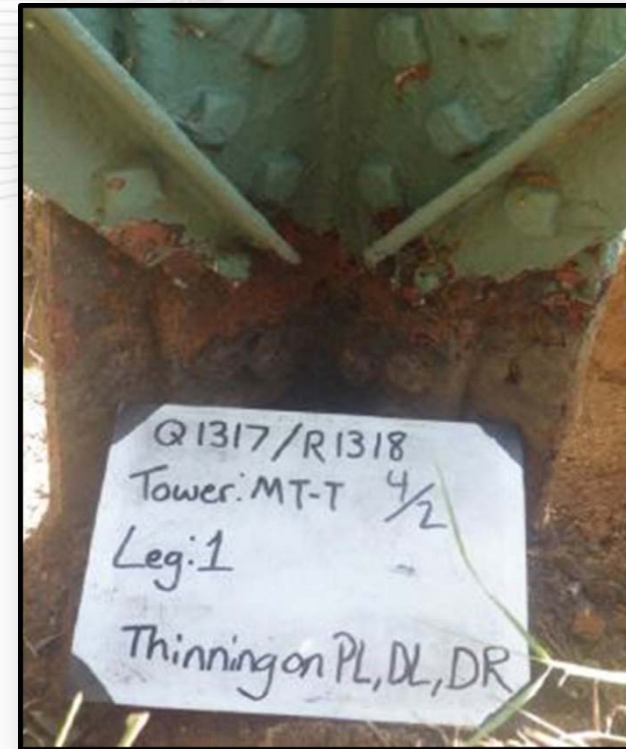
Figure 1: Examples of 25-30% foundation structure loss
