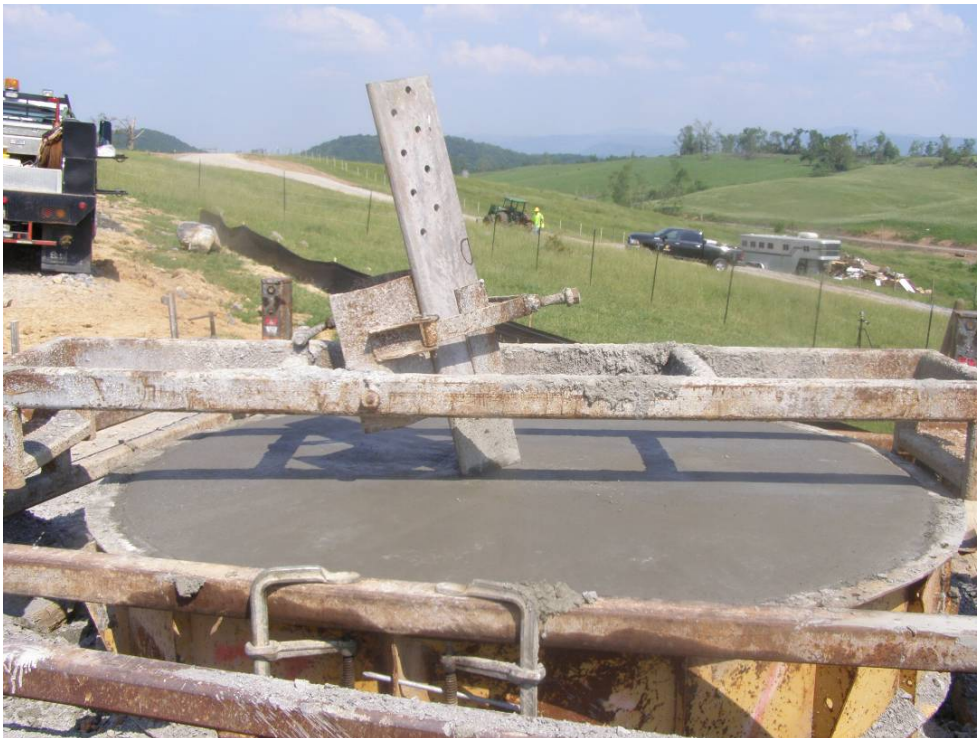
Figure 6 – Concrete Form with Stub Jack and Positioner
