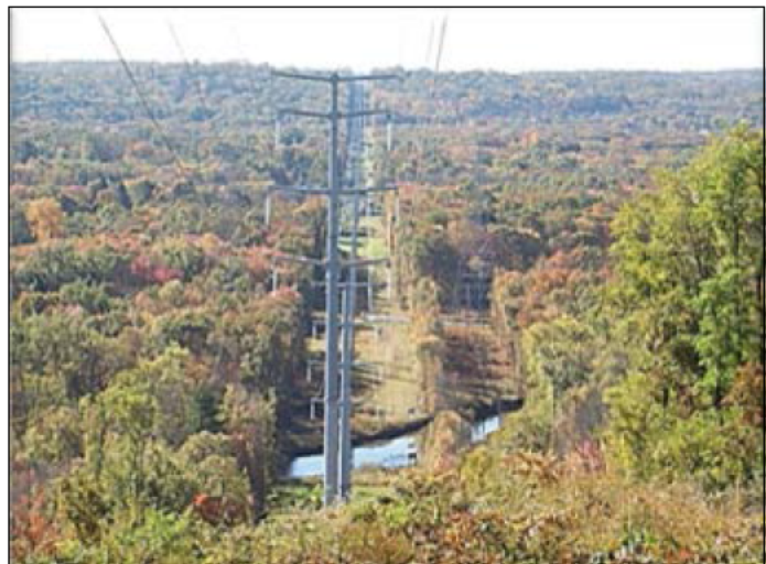
North Central Reliability Project
